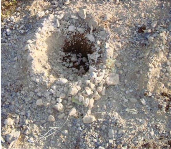
4. A, B If your soil is dry, some soil might collapse in the freshly dug hole. Just use post hole digger to get the soil out of the hole.
