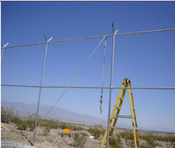
28. A, B: Once the cage frame was finished, with all the poles and top, middle and bottom rails in place, it was time to hang the chain link, using ladders and different tie downs and winch straps to get it up to the 12 feet height.
