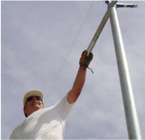
27. Attaching top rail sleeve to the top rail, following the string attached to poles, which is used as a guide to make sure all is in the straight line.
