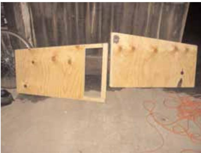
Left and right walls with sheathing in place. Nowhere is the polystyrene exposed to the cats. See door?
