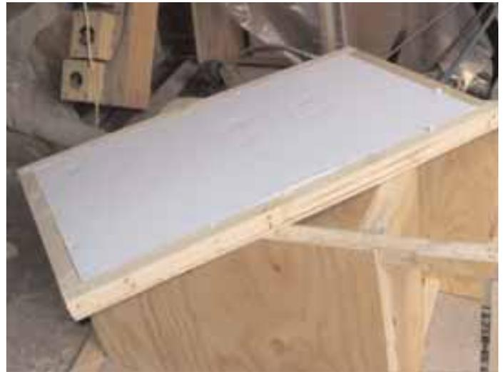
...filled with foam. Plywood sheathing covers both sides. I recommend covering the floor with linoleum.
